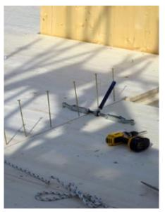
Self-drill woodscrews installed using lightweight power drivers.
