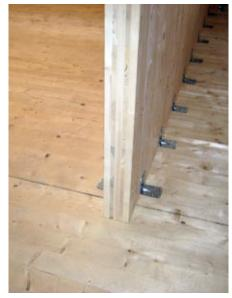
Wall panel anchored to floor panel.
